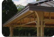
**Options Shown:** Standing Seam Steel Roof, 2x6 Tongue & Groove Roof Decking, Steel Posts & Beams, Ornamental Railings and "J" style Fascia, 40 lb. Snow Load
