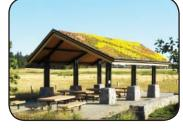
**Roof Style:** Ship Prow Extensions at Gable **Options Shown:** EcoRoof, Double 6x6 by 3/16" Steel Posts, \*Stone Facade (by others)
